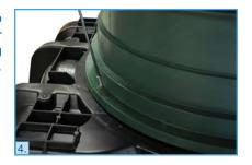
5. Complete with the riser and lid installation and backfill as specified in the Infiltrator Systems, IMand TW-Series Septic Tank Riser Connection Guidance. Backfill per tank manufacturer's instructions.
